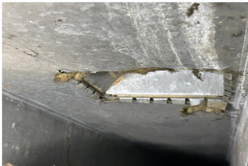
Re-Connect & Seal Leaky Duct Connections
