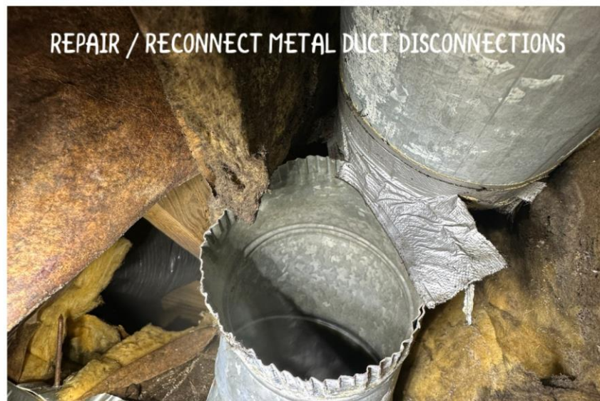
REPLACE METAL DUCT CONNECTIONS OR COMPONENTS THAT HAVE FAILED AND ARE UNREPAIRABLE
