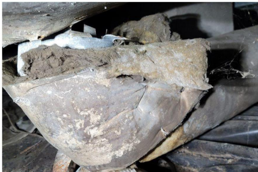
Re-Connect & Seal Leaky Duct Connections
