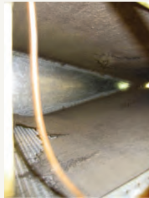
Fouled Coil: This photo shows the upstream side of a heavily-fouled A-coil, which is essentially matted over with dust and other contaminants.
